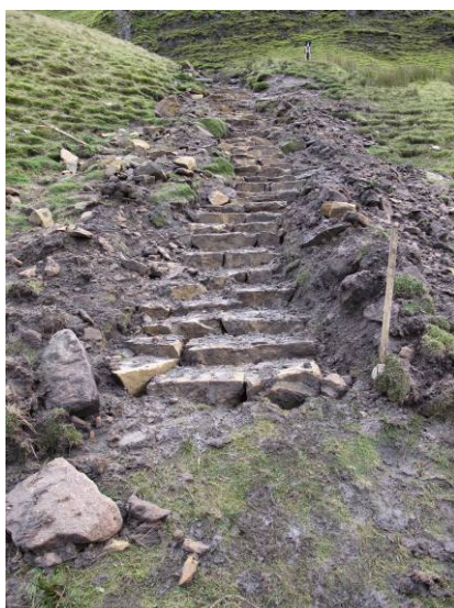
Stone Pitching in Progress, Plover Hill, Pen Y Ghent
