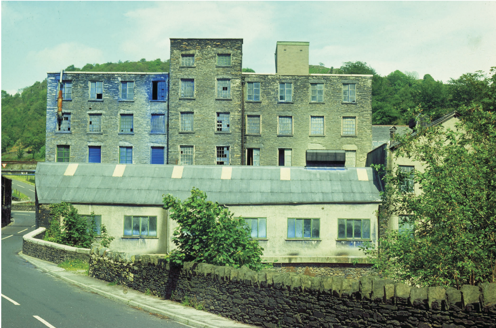
Ultramarine Blueworks, 1980s Note the blue stains around the windows on the left
