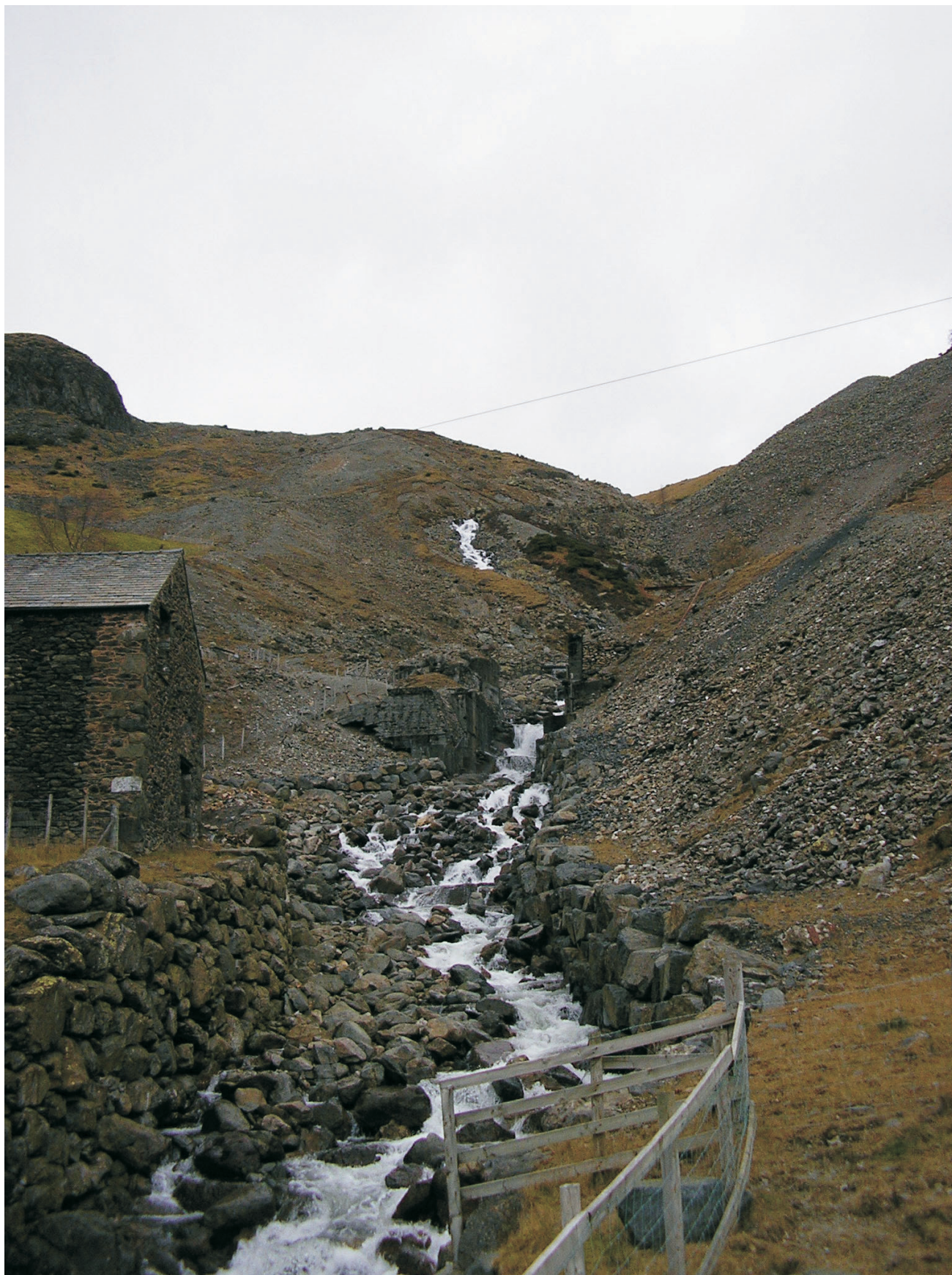
Swart Beck – a power source and washing facility for Greenside Mine
